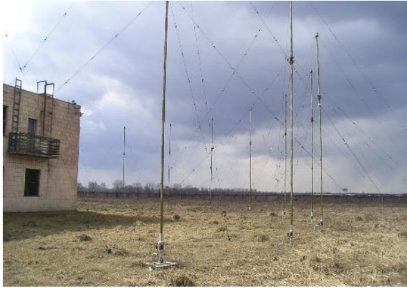
General view of “R-700M” RDF station layout
