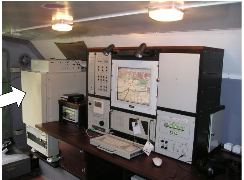
View of operator workplace of "Ukol-RK" station
