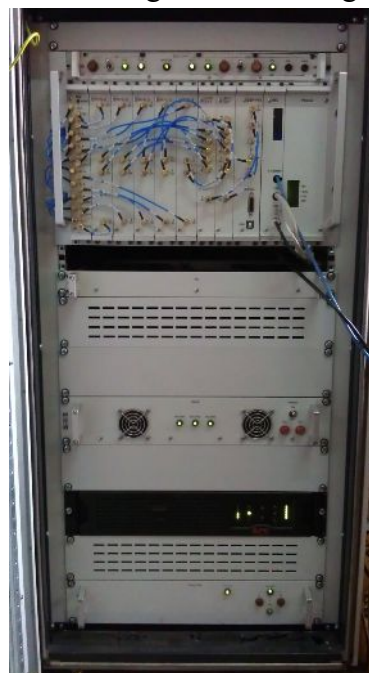
Rack of receiving and measuring device
